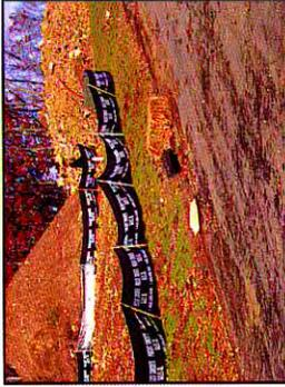
A simple tarp over this stock pile and geotextiles can help to avoid this problem.
