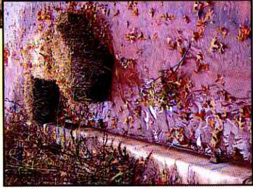
Maintain erosion controls for the duration of the project. Geotextiles, filter fabrics and gravel are all excellent sediment controls (BMPs), however regular maintenance is essential.
