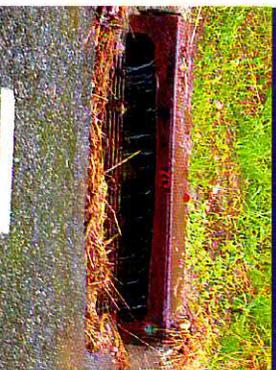
Stormwater can pick up sediment, debris and other pollutants as it runs off and enters nearby stormdrains.
