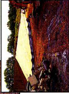
Geotextile/silt fence used to stabilize bank erosion.
