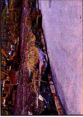
Exposed stock piles and soil can easily run off construction sites resulting in costly repairs clogging drainage structures.
